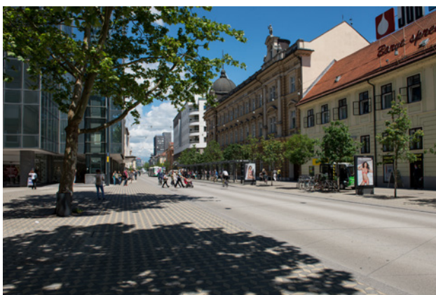
One of the city centre renovation projects in the City of Ljubljana Author: Doris Kordić
